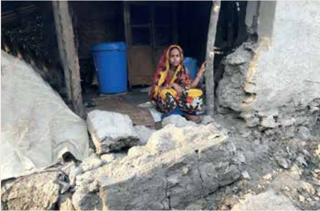
Figure 01: A House Destroyed by Cyclone Remal
