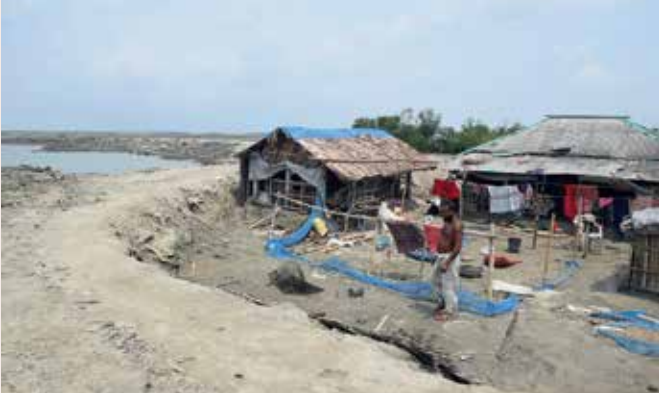
Figure 03: Fragile Embankments are Risky Homes
