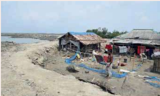
Figure 03: Fragile Embankments are Risky Homes
